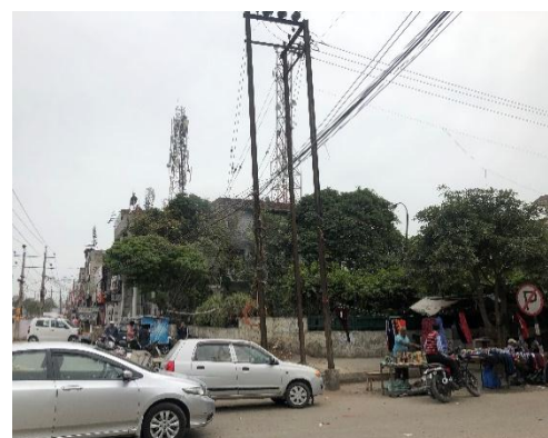
Figure 20: Carriage way encroached by buyers at Rishi Nagar road Source: Primary Survey
